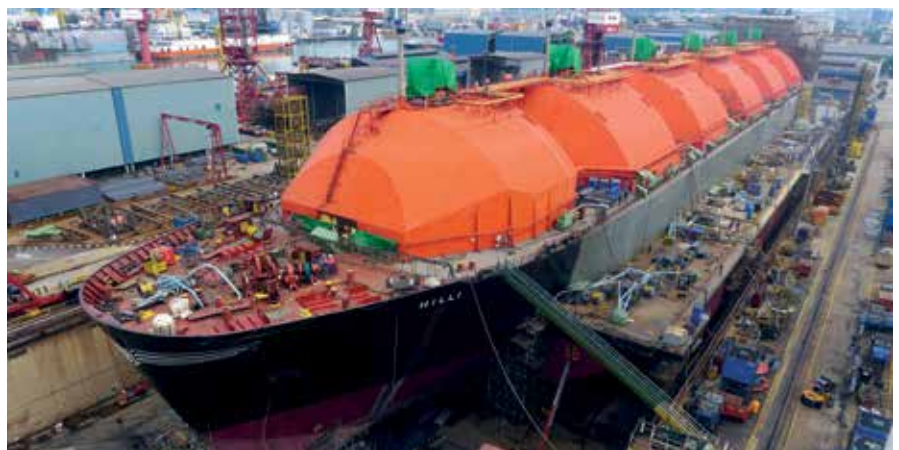
The conversion of LNG Carrier, Hilli, by Keppel Shipyard into an FLNG vessel is progressing well and is about 68% completed to date
