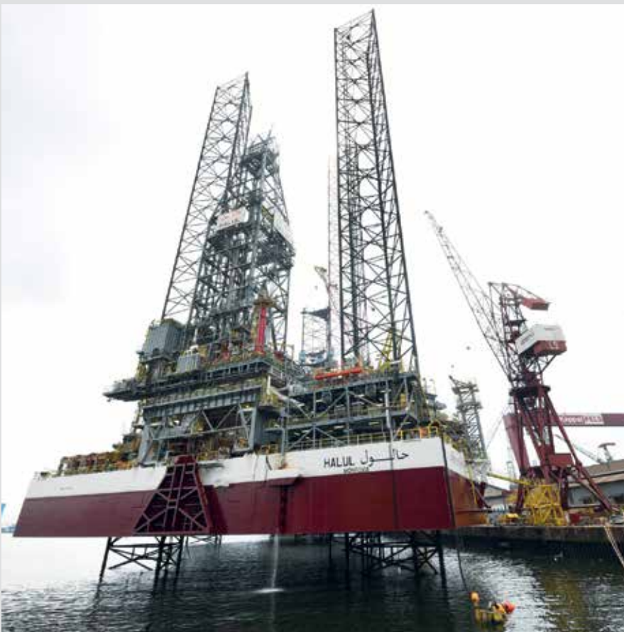
Halul was completed 10 days ahead of schedule, on budget and with a perfect safety record. It will be the fifth KFELS B Class jackup rig to work for Gulf Drilling International
