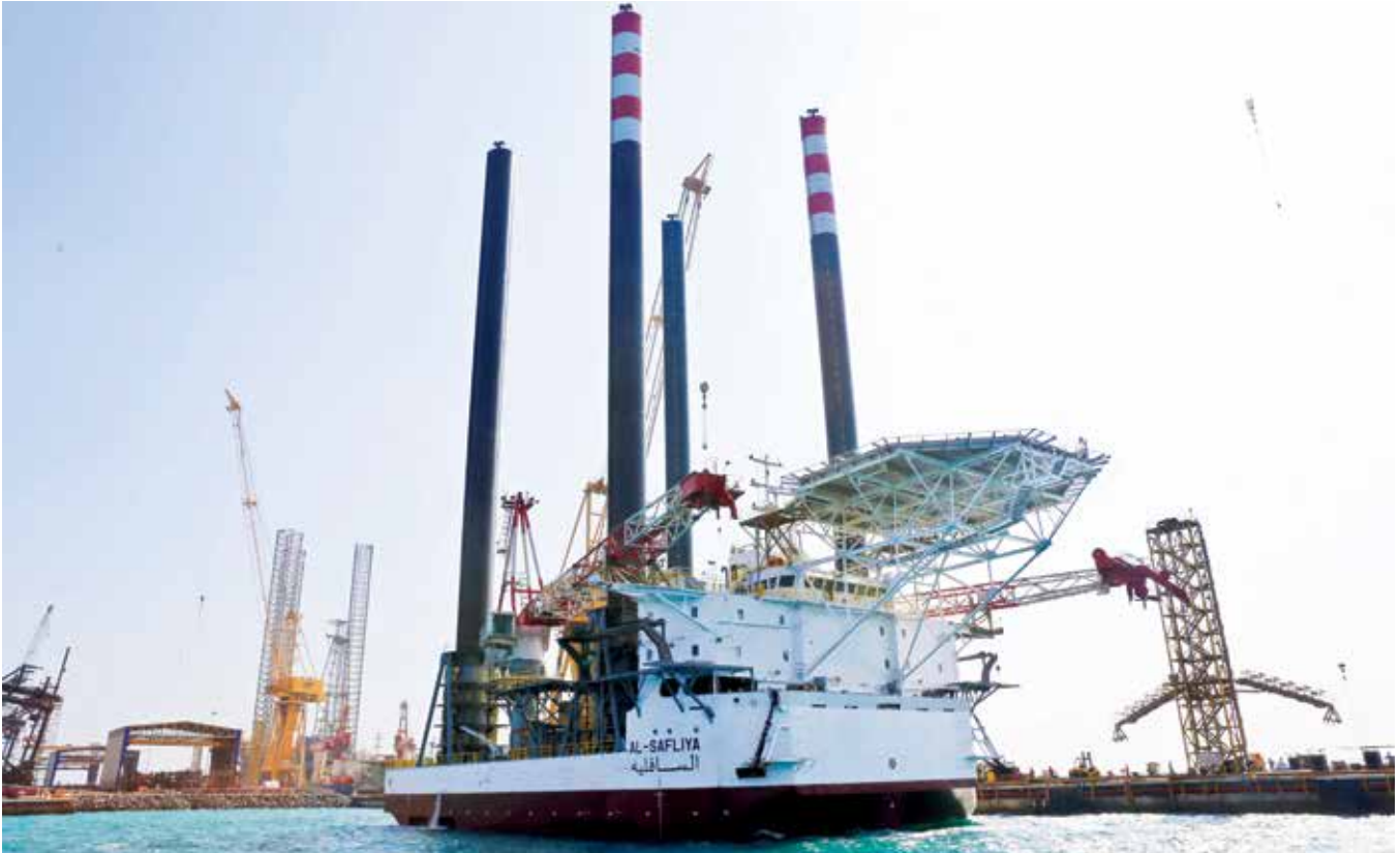
Al Safliya, the first liftboat to be wholly constructed in Qatar, is built to the ORCA 2500 design developed by Keppel O&M's design arm, Bennett Offshore
